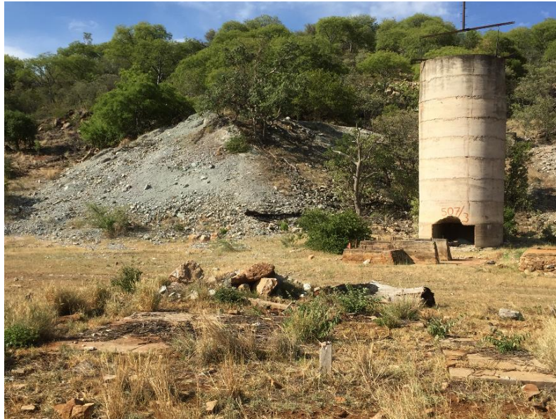
Deblin Mine silo, waste-dump and remains of infrastructure
