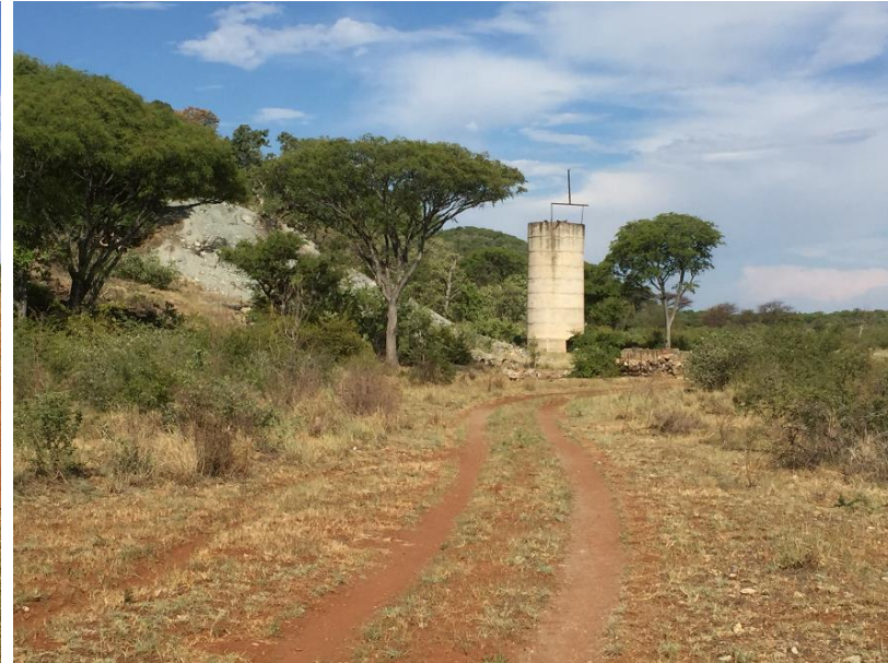
Access track south of Deblin Mine Ridge, showing ore silo and waste dump
