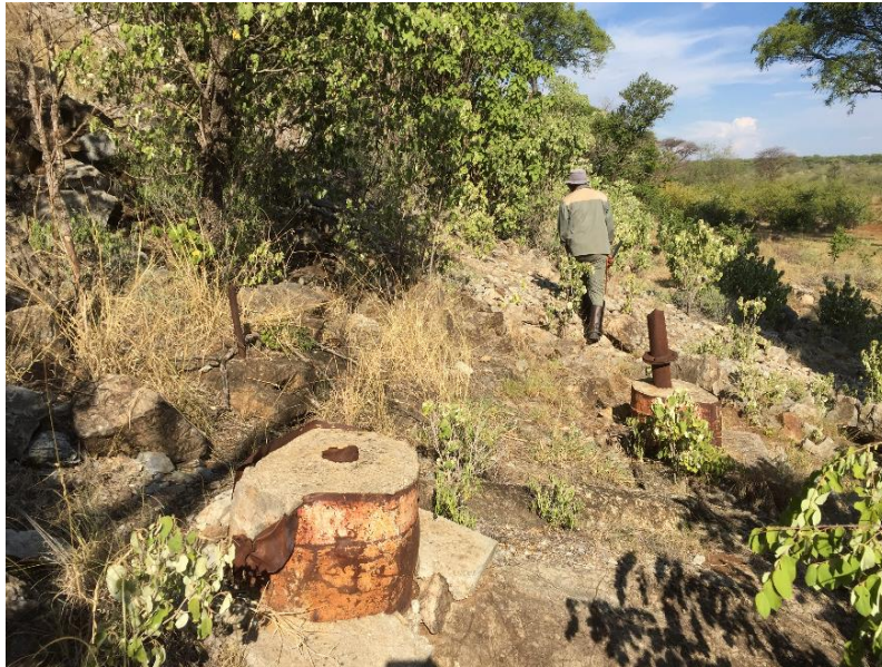
Deblin Mine -foundations of conveyor system pillars
