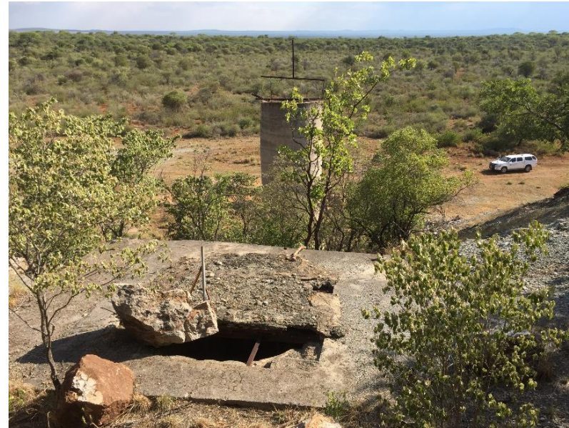
Deblin Mine shaft (foreground) and ore silo (background), vehicle for scale
