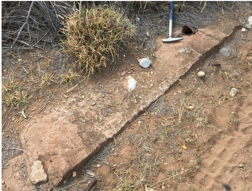
Old drill-site foundation, concrete drill-pad with anchors and uncapped standpipe (1970's)
