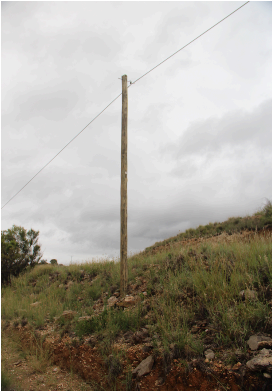
Figure 3 - Low impact installation of poles (existing Paratus project – status complete)
