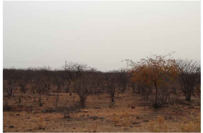
Figure 12 – Overhead line and local vegetation
