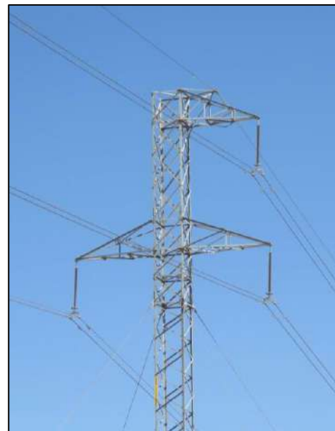
Figure 3 a, b, c. Examples of the guyed lattice steel pylon structure that will be used for the proposed 220 kV B2Gold power line; the design is single circuit, with three conductors and one additional optical ground wire (OPGW or earth wire) running at the top of the configuration (F de Wet pers. comm.).
