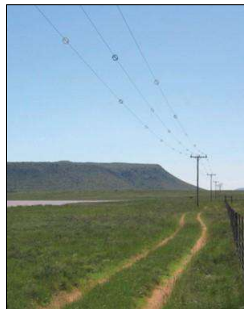
Figure 35. Example of a SWAN-FLIGHT Diverter (SFD; made by Preformed Line Products [PLP]), as a mitigation for bird collisions.
