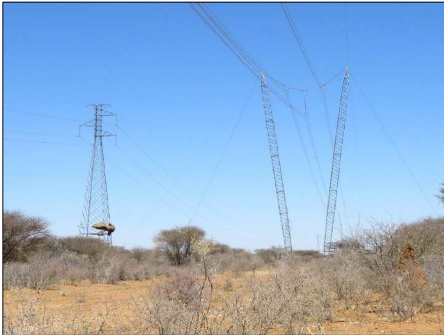
Figure 6. The existing NamPower 220 kV Gerus-Otjikoto line (No. 1 and 2) on Farm Maxwell (looking south-westwards), consisting of a self-support steel lattice structure (left) and a guyed-V structure (right). Note the large Sociable Weaver nest on the left-hand tower.
