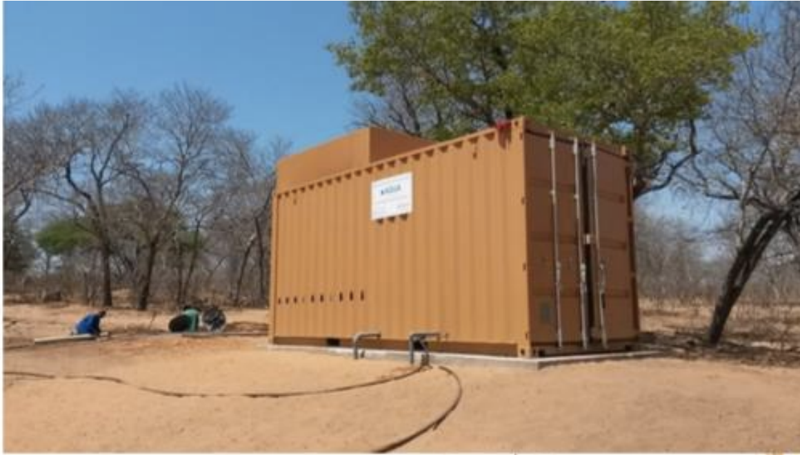
FIGURE 3 - TYPICAL CONTAINERISED SEWERAGE (TRICKLING) TREATMENT PLANT.
