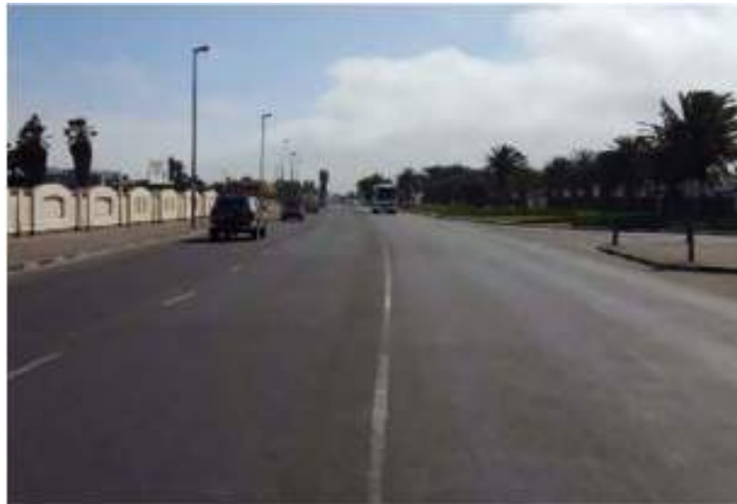
Photo 15: South-Westbound View along Nangolo Mbumba at Esplanade Str
