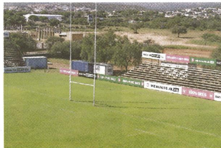
EVAMPED: The Hage Geingob Rugby Stadium after renovations. Photo contributed
