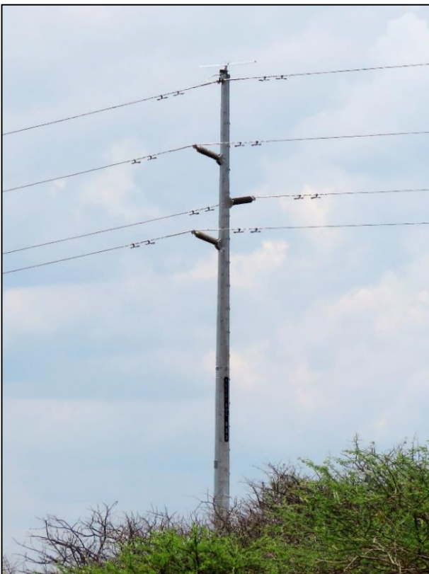
Figure 4. Examples of the proposed self-supporting steel monopole structure for the 66 kV power line, showing structure at a bend point, with stay wires (top left & right; photos F de Wet); and configuration of conductors with optical ground wire (OPGW) above, topped by steel perching device as a mitigation for electrocutions.
