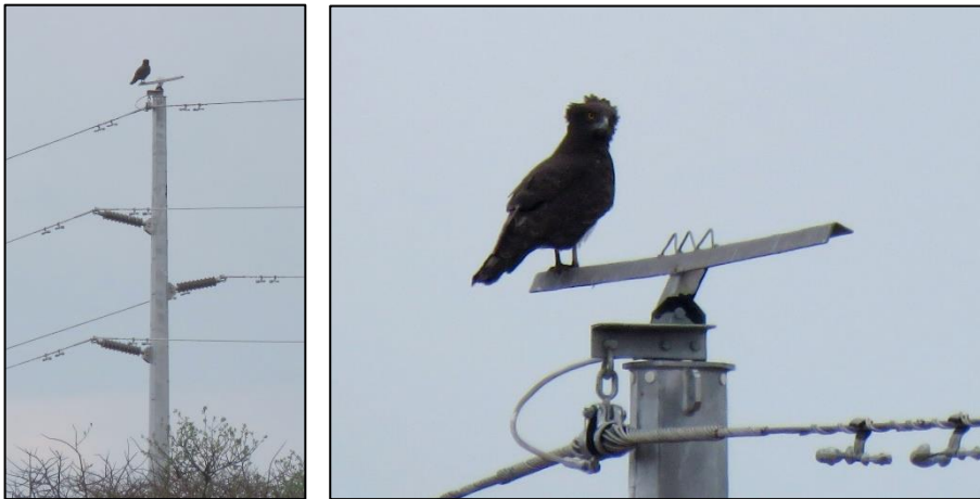
Figure 26. Example of use of a perching structure fitted as a mitigation for electrocutions to the 66 kV Eldorado-B2Gold steel monopole structure by a Brown Snake-eagle.
