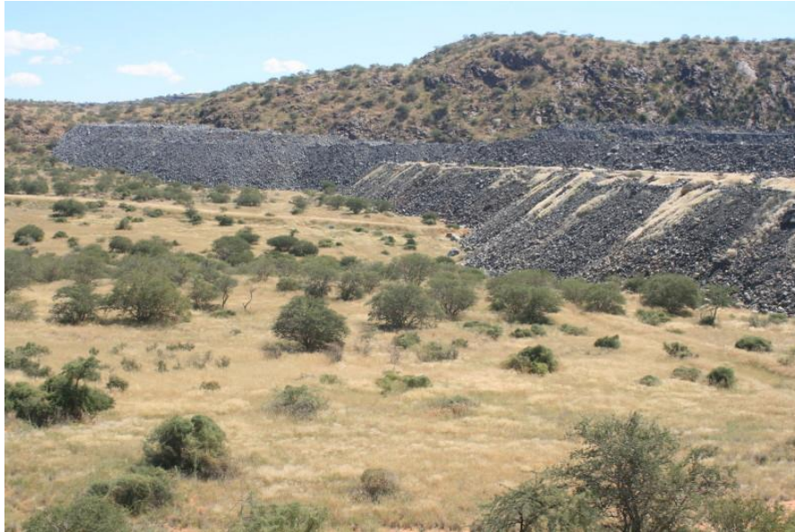
Figure 27. The TSF3 rock bunding walls should be covered with soil to facilitate vegetation regrowth and not left as bare bedrock. Note the limited, albeit natural, grass establishment in areas where some soil had accumulated over time.
