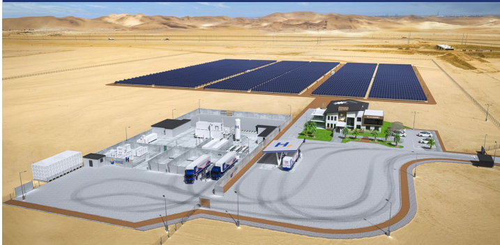
Experience with hydrogen & ammonia
