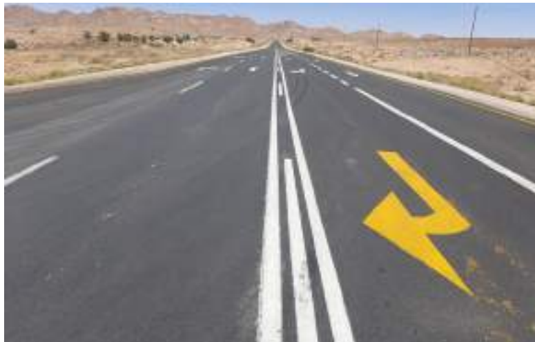
Photo 3: Westbound view along the B4 from the C13 / B4 intersection
