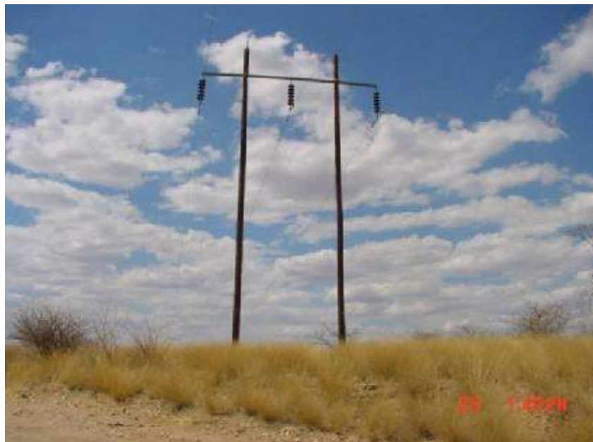
Figure 3: Wooden H-pole design.
