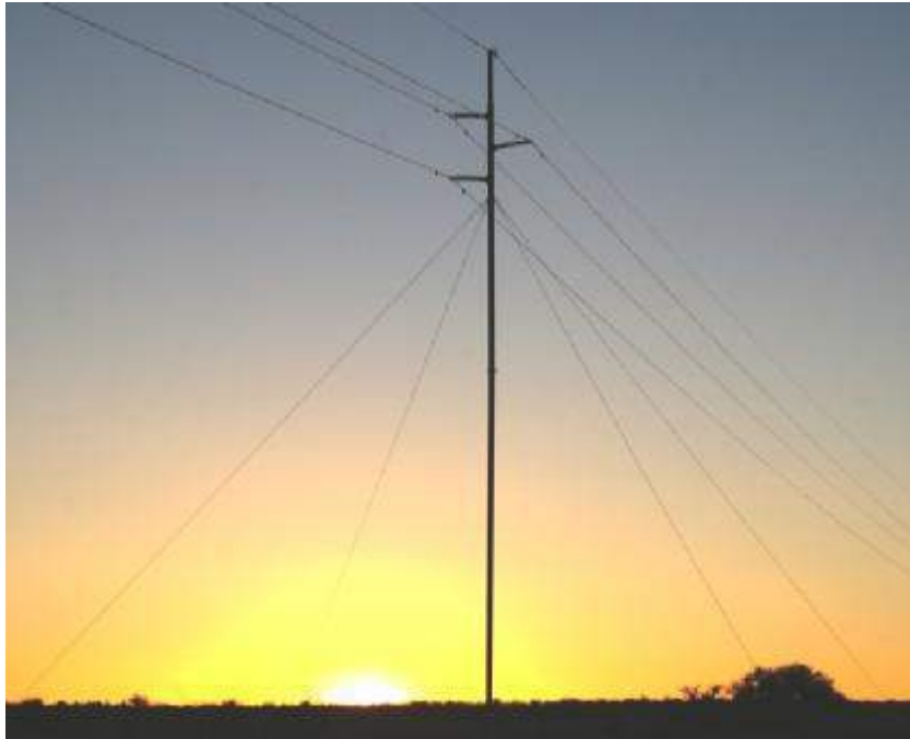
Figure 4 Steel monopole design.
