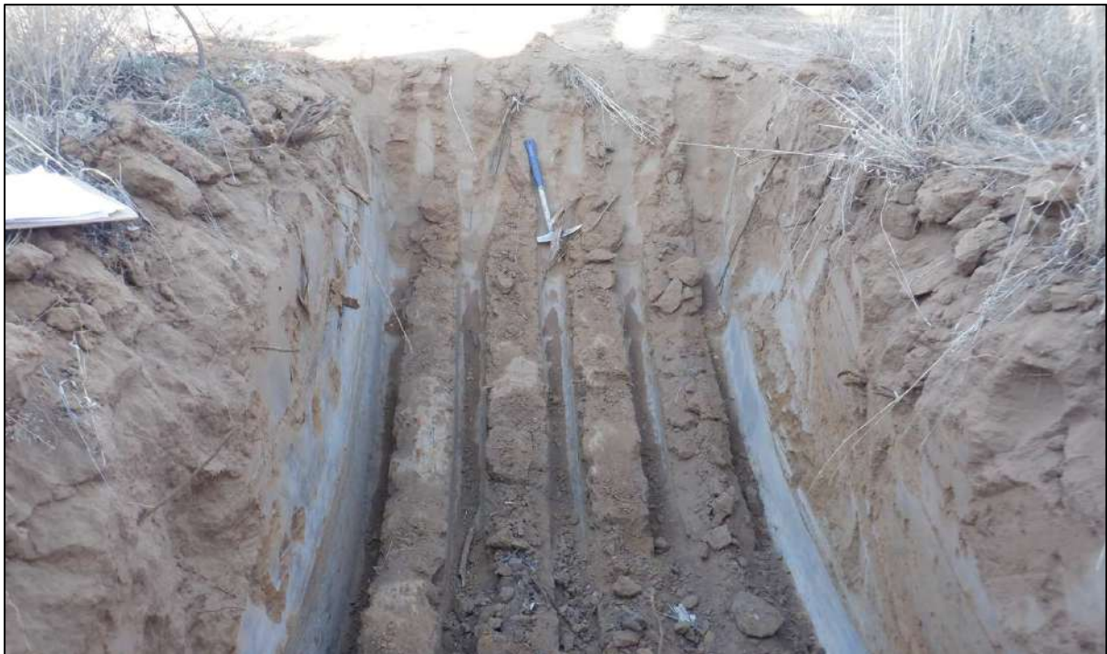
Plate 12: Shallow excavator refusal on ferruginized alluvium at HLP-TP28.
