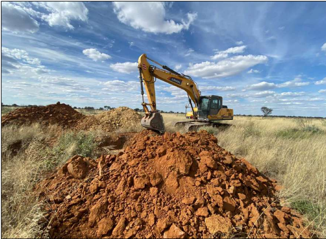
Plate 3: Northerly view of excavations underway at SWD-TP11.
