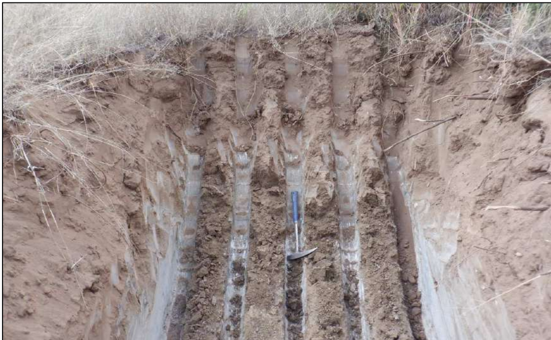
Plate 2: Shallow excavator refusal at SWD-TP08 on ferruginized alluvium of soft rock strength.
