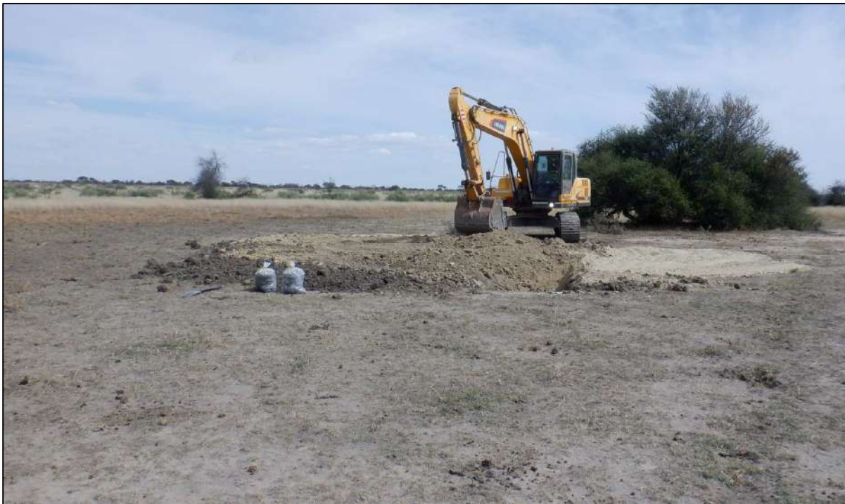
Plate 6: Rehabilitation of SWD-TP26 within low-lying clay pans.
