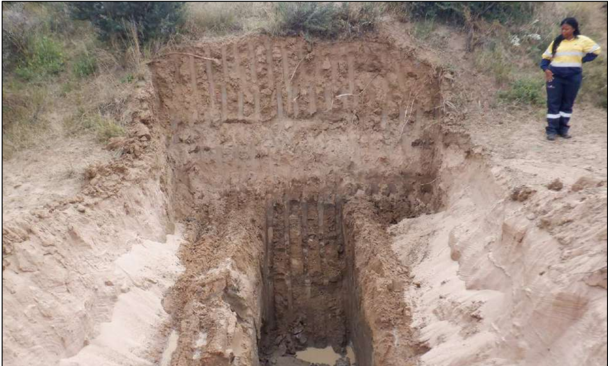
Plate 13: View of soil profile and shallow water table at WRD-TP01.
