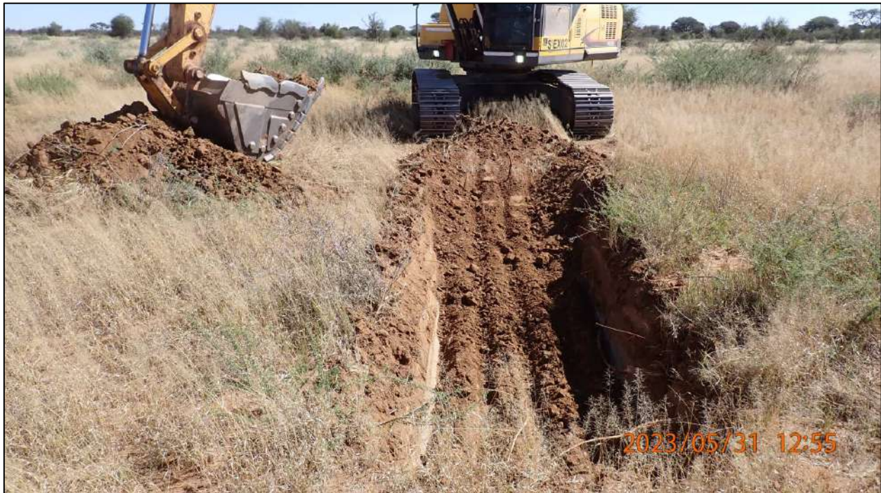
Plate 28: Excavations underway at AM-TP01.
