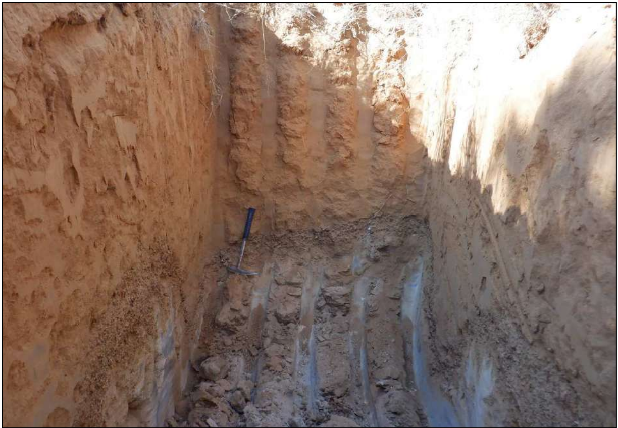
Plate 11: Typical soil profile at HLP-TP26.
