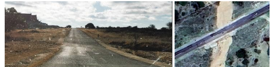
Photos at km 7.1, MR 59, sealed concrete drift
