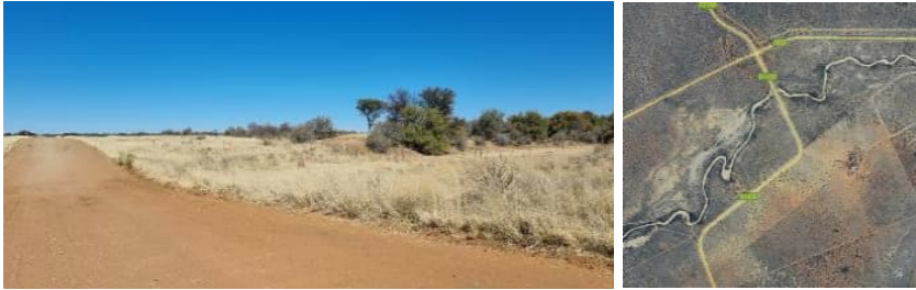
Photos of water course crossing on DR1435 at km 48.6
