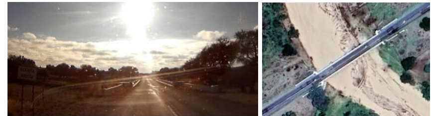
Photos at km 2.8, MR 59, stormwater structure: 5.8m wide
