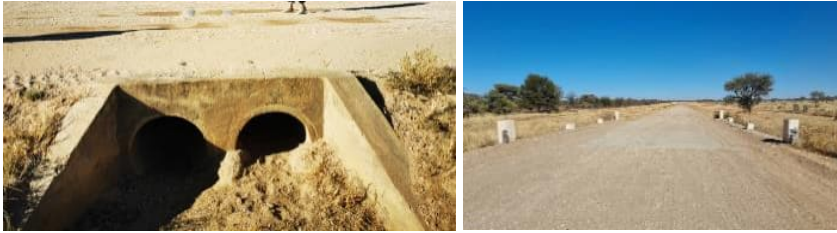
Photos of stormwater structures on km 42.8, MR 59 and km 12.4, MR60.
