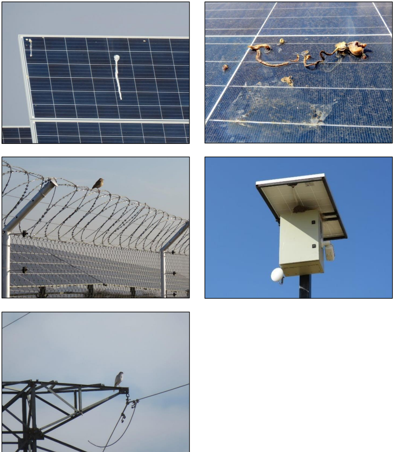
Figure 14 a-e. The infrastructure associated with the existing solar PV plant has created further artificial habitats that are used by birds for perching, feeding and nesting opportunities: evidence of bird perching on the panels (a) and of feeding on prey on the panels (b); African Pipit perching on security fencing (c); Rock Martin nest on security structure (d); Pale Chanting Goshawk perching on power line structure (e).
