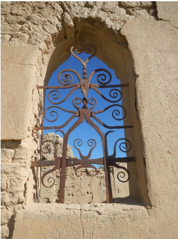
Figure 7: Okawayo 480, detail of wrought iron window bars.
