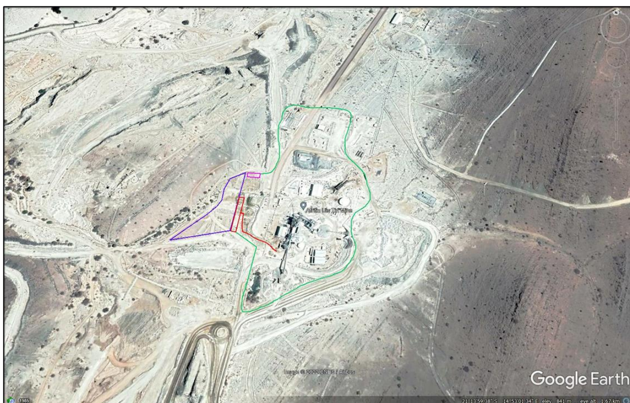
Figure 19 - Uis Tin Mine with the indicated infrastructure upgrades required for Phase II. Green indicates the impact area for future operations. Pink indicates the new sewage plant (Bio-Mite). Purple indicates the newly planned water return pond. Red indicates the newly planned settling pond and canal (Source: Uis Tin Mining Company (Pty) Ltd).
