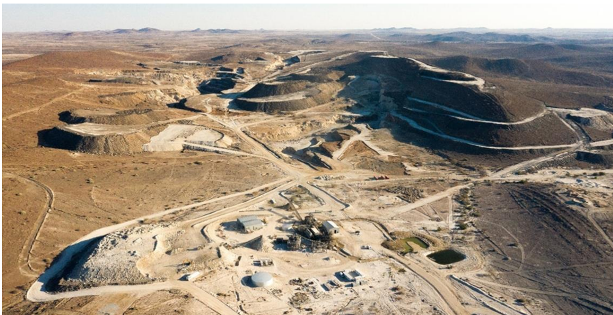
Figure 12 - UTM Mine and Ore Processing Infrastructure (Source: Minxcon, 2020)
