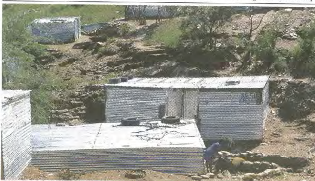
DANGER: Shacks built in riverbeds.
