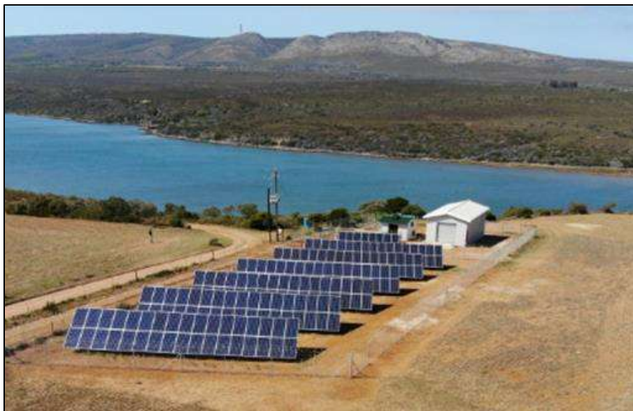
Figure 6. Typical solar photovoltaic panel array at the Witsand Solar Desalination Plant in South Africa ( https://www.osmosunwater.solutions/en/project/osmosun-16-sw-witsand-solar-desalination-south-africa/ ; http://www.hessequa.gov.za/witsand-solar-desalination-plant/ )
