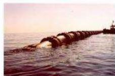
Fig 0.2.2.5 The submerging process has started 2020/06/08
