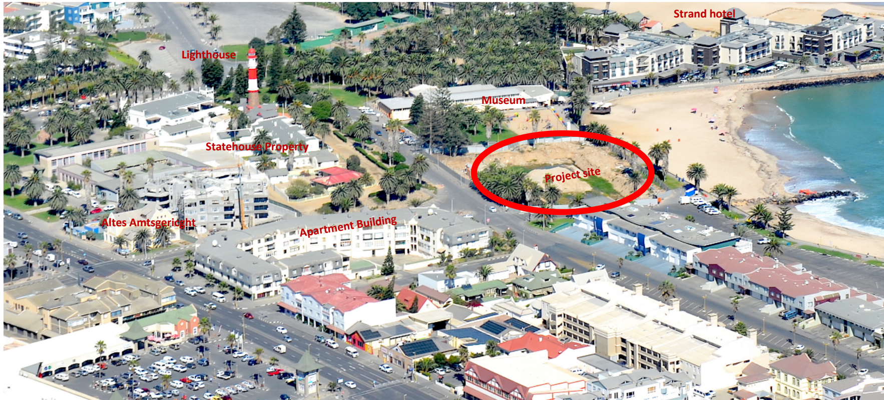
FIGURE 17 - AERIAL VIEW NORTH-EAST FROM ERF 4747
