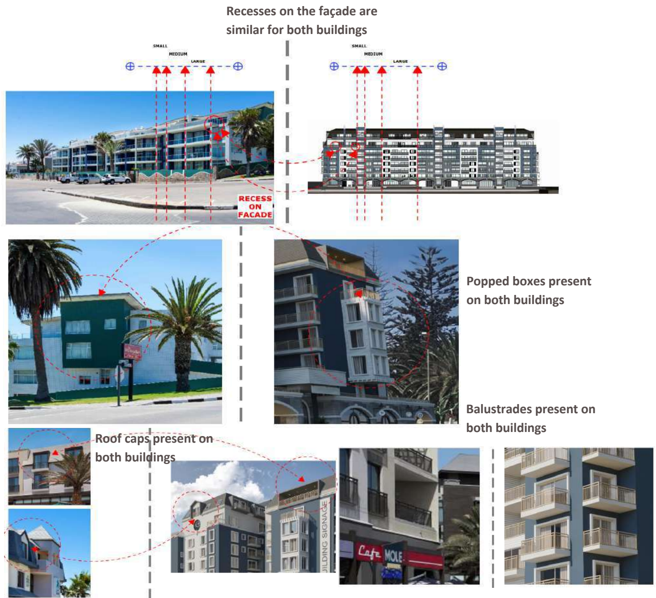
FIGURE 13 - OTHER DESIGN COMPONENTS OF THE BUILDING
