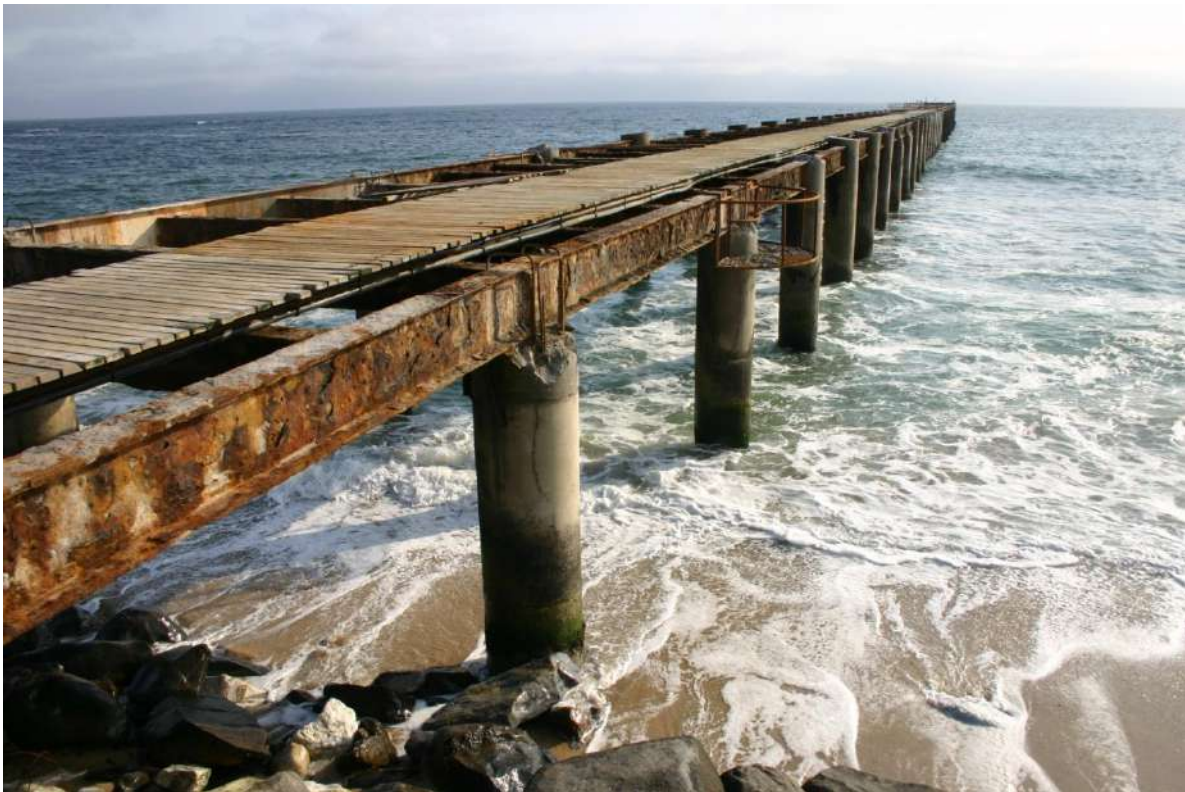
The steel jetty after restoration in 1998
