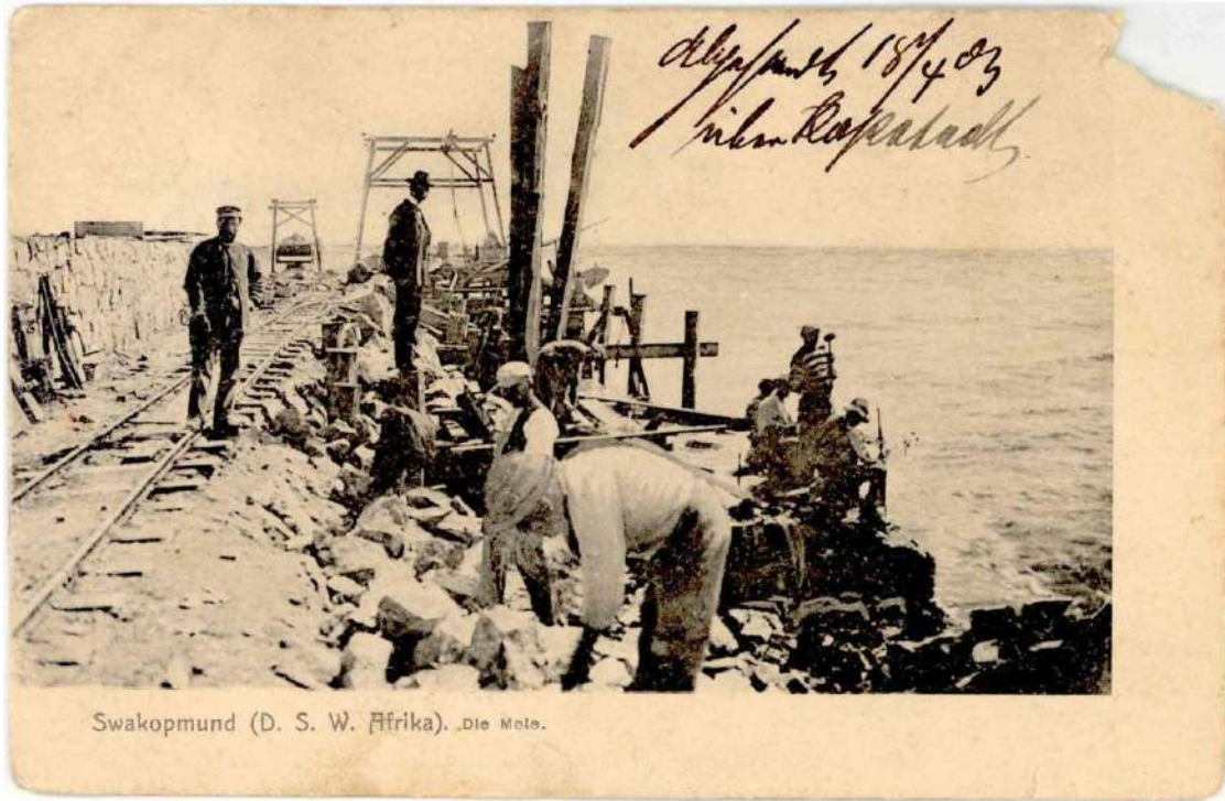
Construction of the harbour mole in 1903
