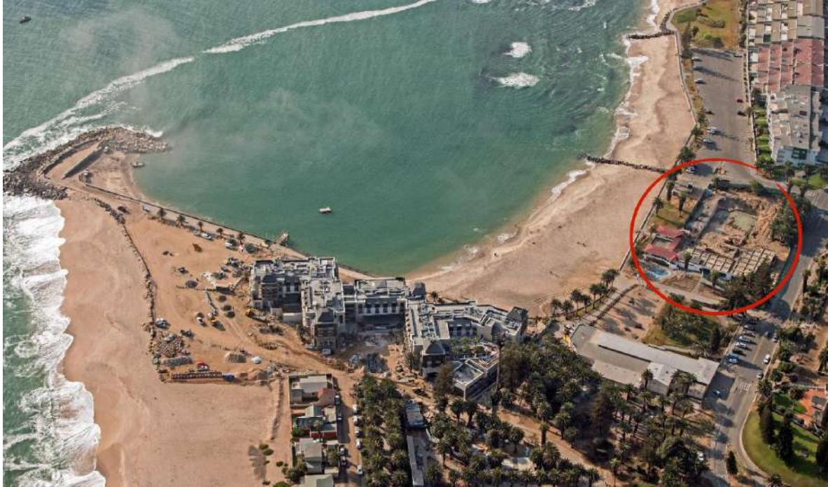
Photograph Courtesy of Lighthouse Property Investment Trust
