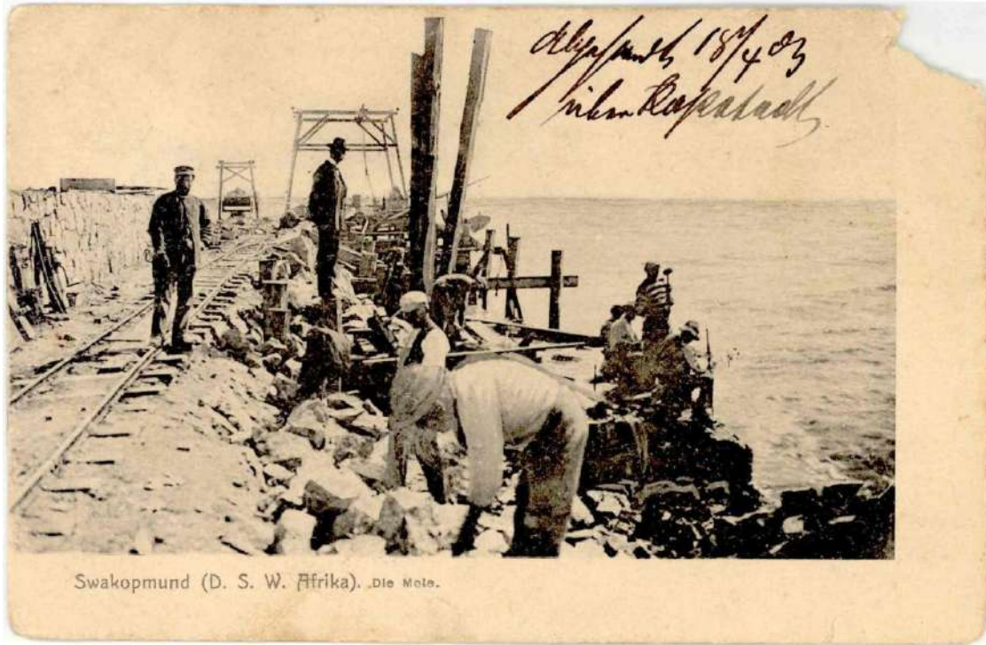
Construction of the harbour mole in 1903
