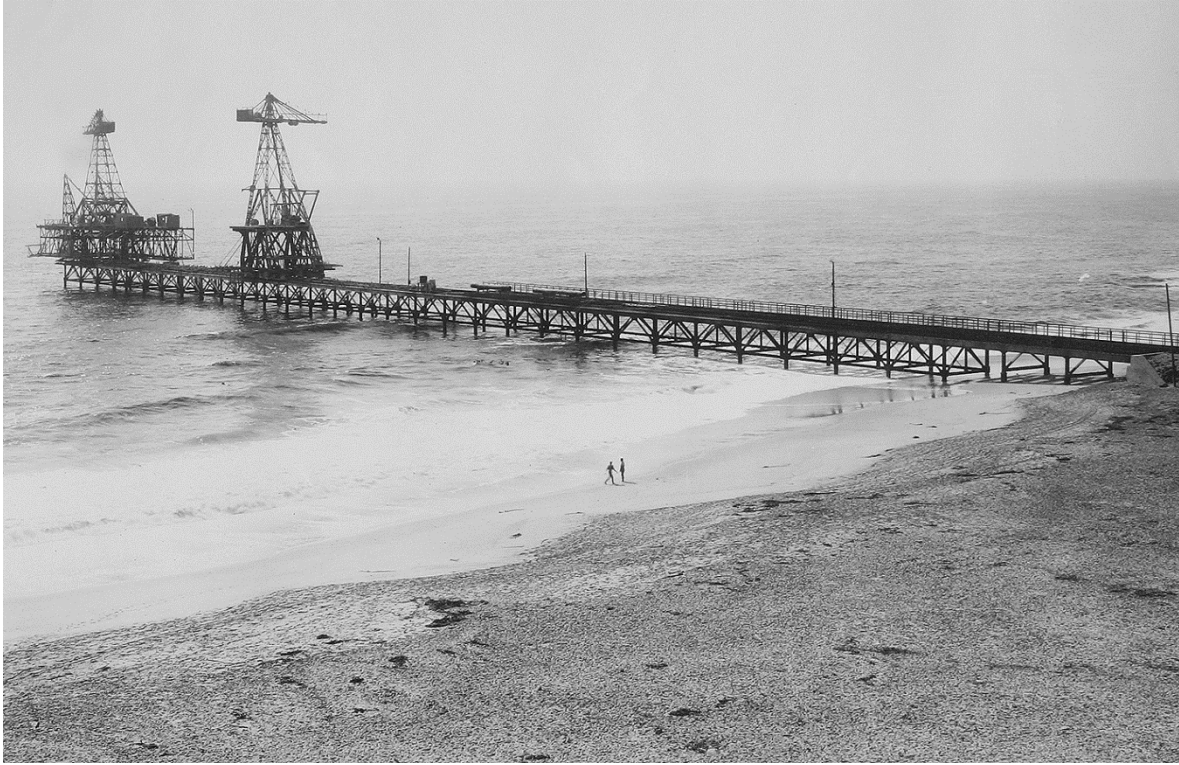
The new steel jetty, built as from 1913, abandoned in 1915 after the war.
