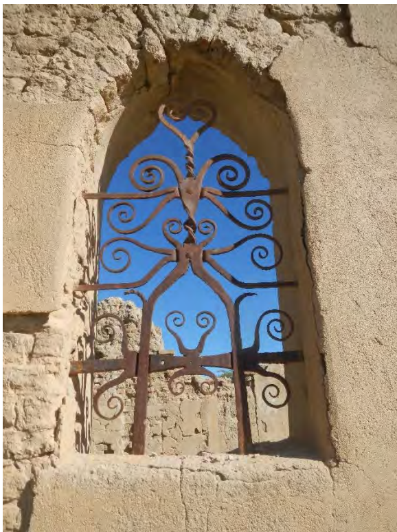
Figure 7: Okawayo 480, detail of wrought iron window bars.
