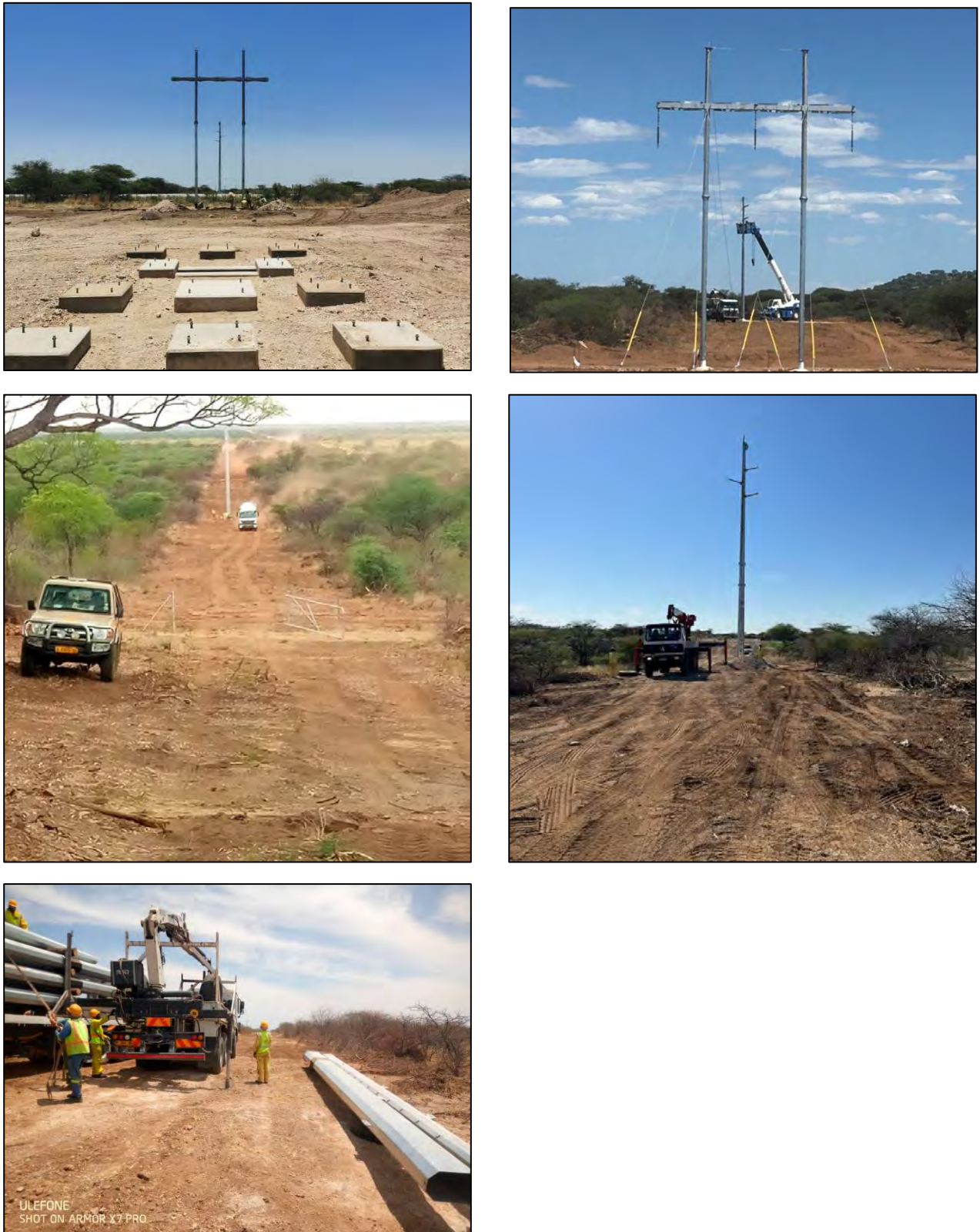
Figure 5. Examples of terminal H-pole structures used at the substation (top left & right); typical construction activities, illustrating the type of disturbance and habitat modification associated with this phase of the project (centre left & right, bottom; photos F de Wet).
