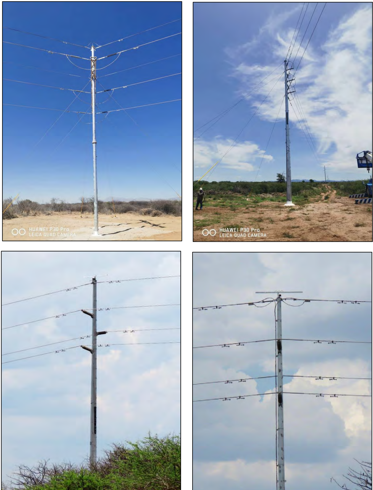
Figure 4. Examples of the proposed self-supporting steel monopole structure for the 66 kV power line, showing structure at a bend point, with stay wires (top left & right; photos F de Wet); and configuration of conductors with optical ground wire (OPGW) above, topped by steel perching device as a mitigation for electrocutions.
