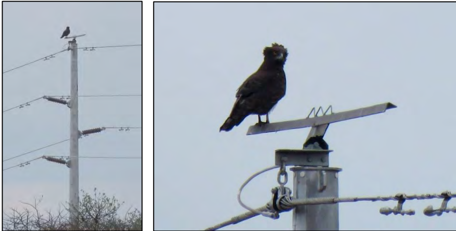
Figure 26. Example of use of a perching structure fitted as a mitigation for electrocutions to the 66 kV Eldorado-B2Gold steel monopole structure by a Brown Snake-eagle.
