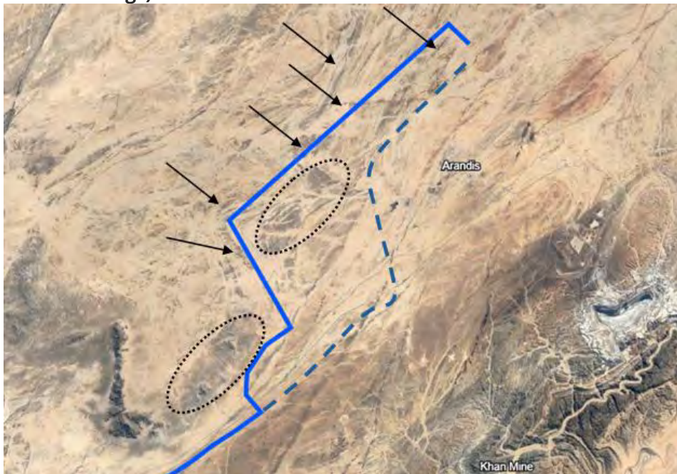
Figure 51 - Arandis pipeline section change (new route being the solid blue line) and associated dolerite ridges (black arrows) and rocky areas (black dotted oblongs)
