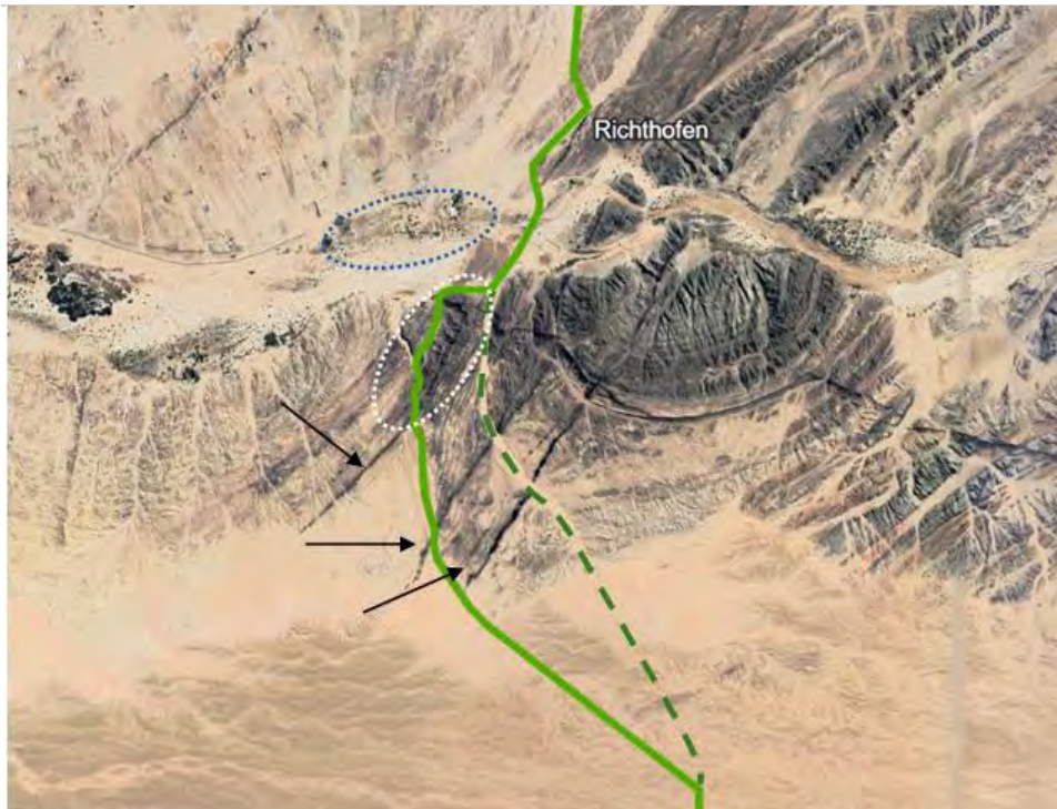
Figure 50 - Pipeline section that crosses the Swakop River (green solid line which is a change from previous dashed route) and associated open surface water and bird habitat (blue dotted oblong); dolerite ridges (black arrows) and rocky areas (white dotted oblongs)
