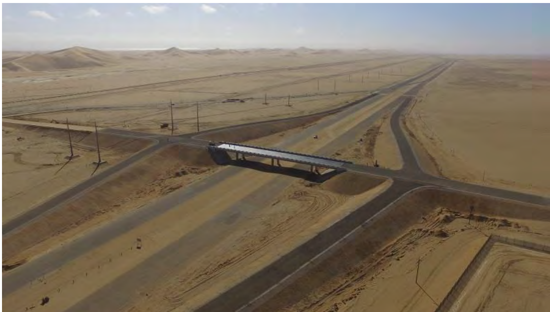
Figure 25 - An intersection-section of the D1987 road (Source: Zutari, 2024)
