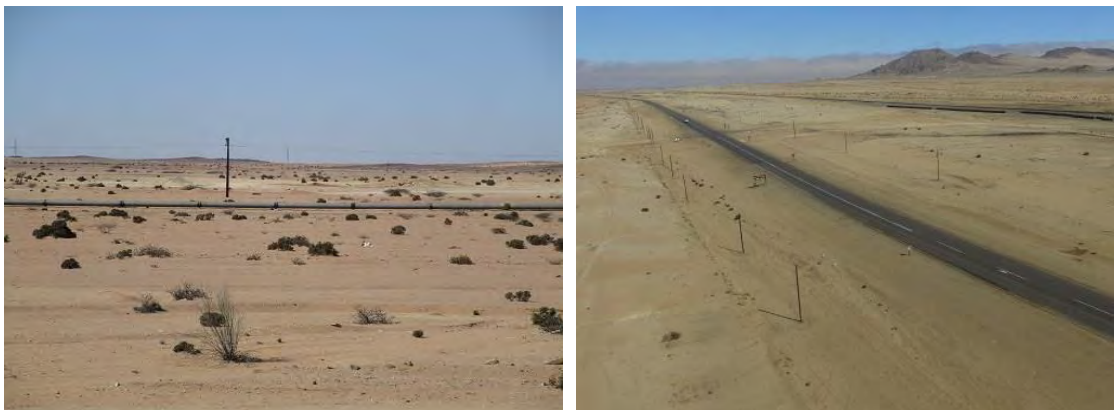
Figure 26 - B2 Main Road crossing between Swakopmund and Arandis (Source: Zutari, 2024)
