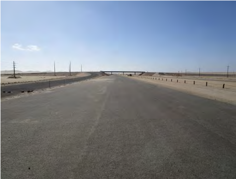
Figure 9 - Photo taken on section of the D1984 Road
