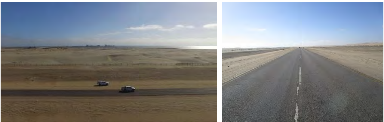
Figure 13 – B2 Main Road crossing at the Ammonia Terminal
