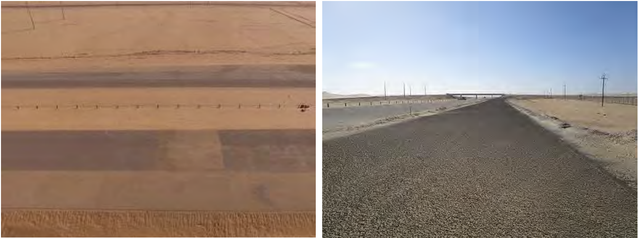
Figure 12 - D1984 Road crossing at the Green Hydrogen Pilot Plant
