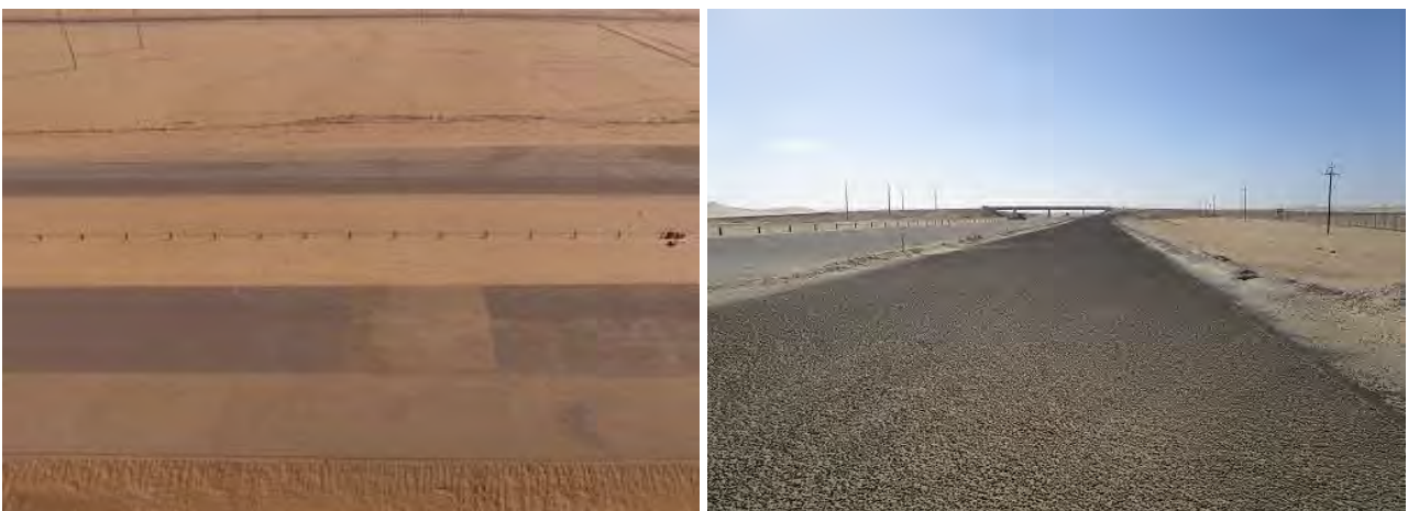
Figure 16 – D1984 Road crossing at the Green hydrogen Pilot Plant Crossing
