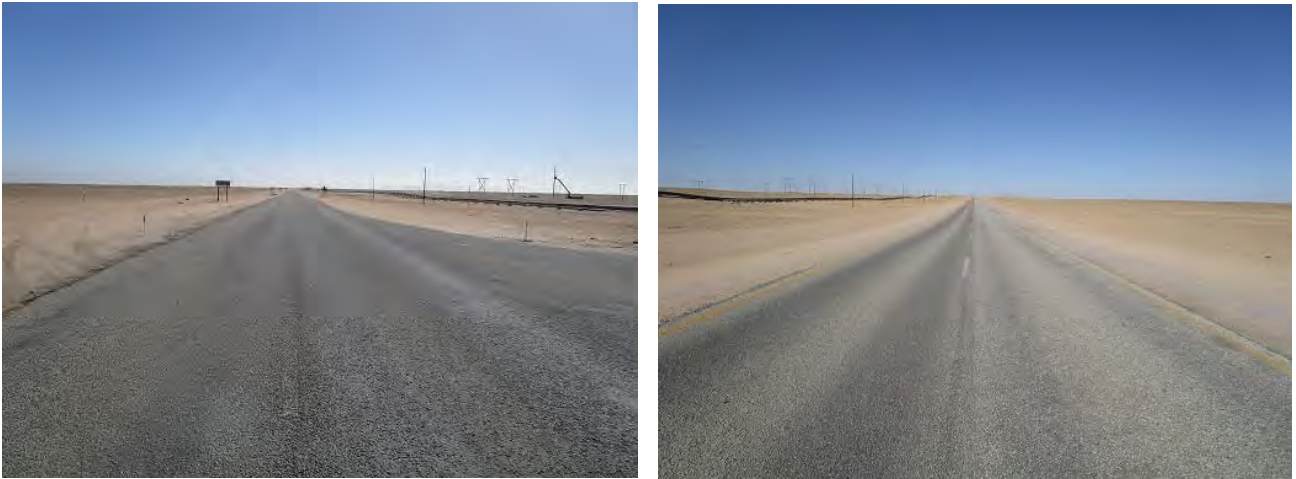
Figure 10 - Photos taken on section of the C28 Road
