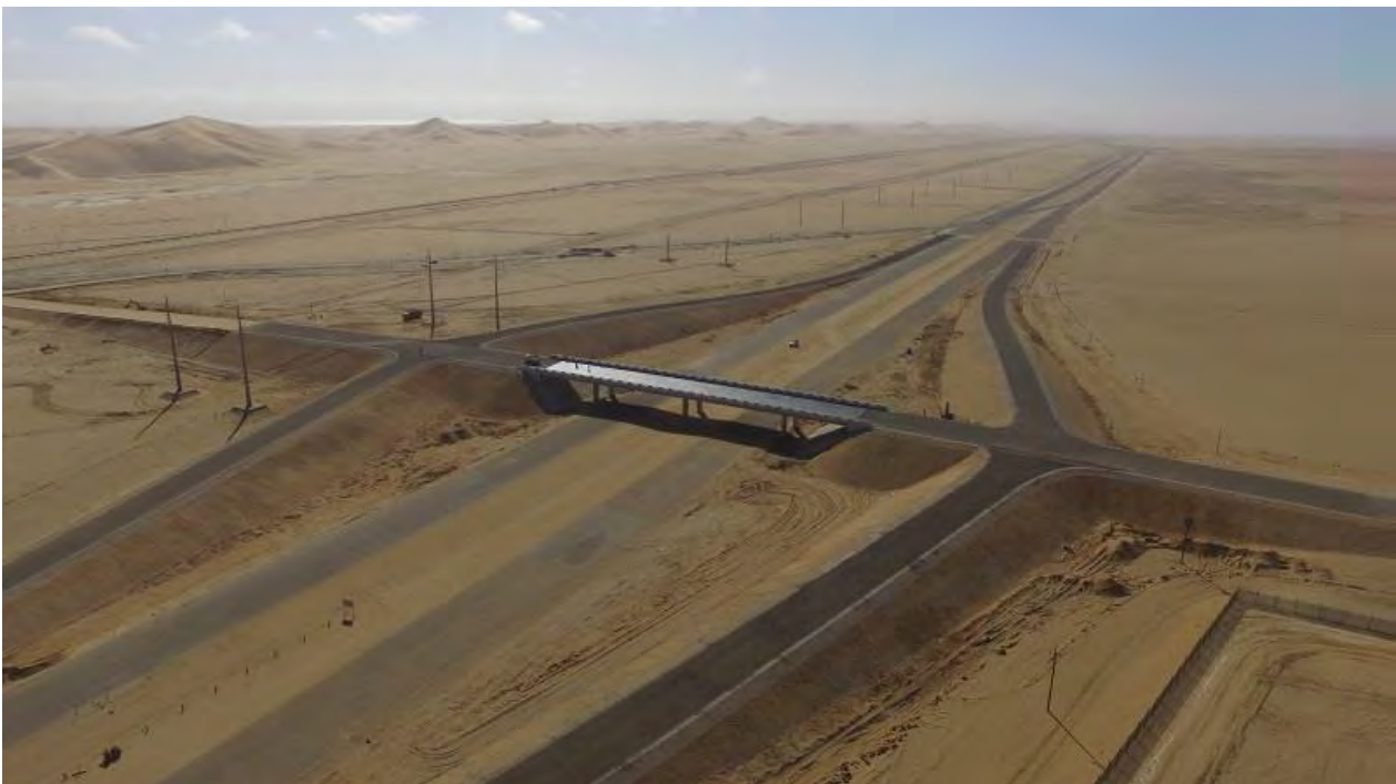
Figure 11 - Photo taken on section of the D1984 Road
