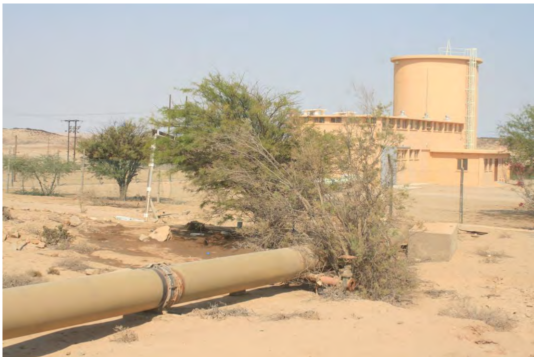
Figure 5. Leakages along the existing water pipeline from Arandis-Swakopmund-Walvis Bay could serve as amphibian habitat.
