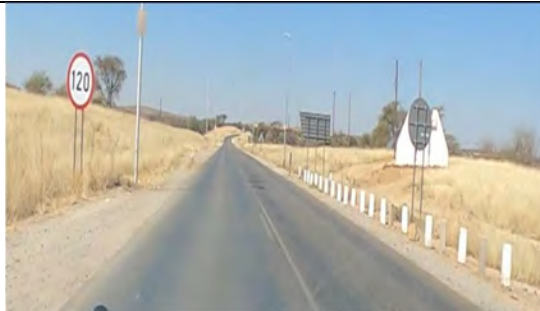
Photo C10: Cross-section of the C33 Road. Northbound view
