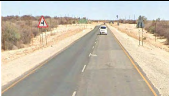
Photo C9: Cross-section of the C33 Road. Southbound View
