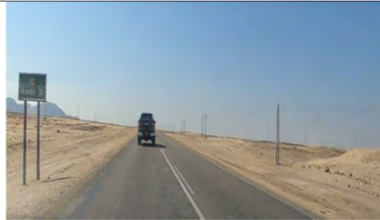
Photo C8: Cross-section of the B2 Road. Northbound View
