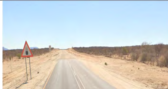
Photo C2: Cross-section of the C36 Road 2km west of the C33/C36 intersection. Westbound View
