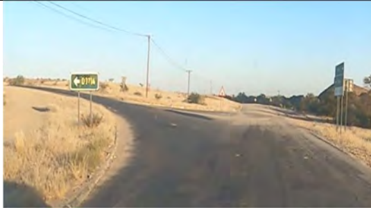
Photo C3: Cross-section of C36 Road at the C36/D3714 intersection. Eastbound View
