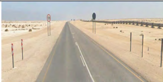
Photo C11: Cross-section of the C34 Road. Northbound view
