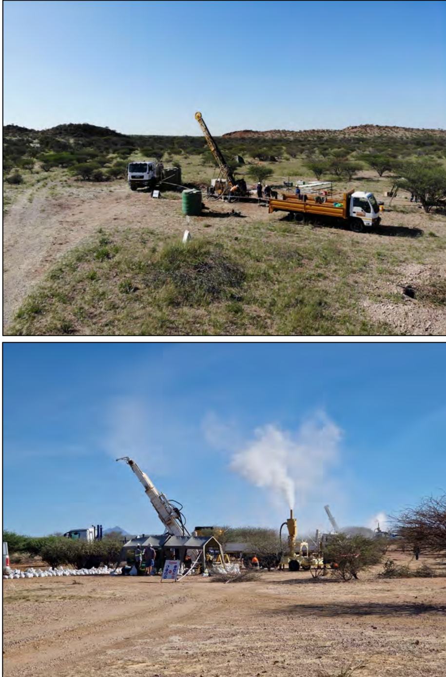
Figure 7 - Images of exploration drilling taking place on EPL 4818 (WiaGold, 2024)
