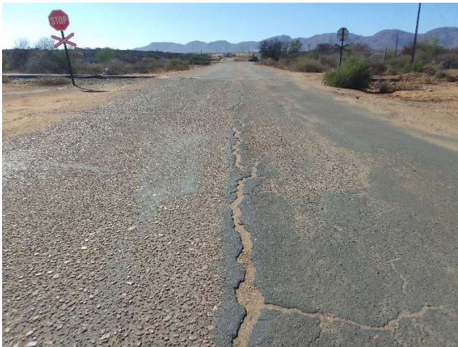
Photo 7: Southbound View along D1527 – Road-Rail Level-Crossing
