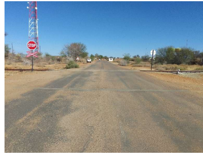
Photo 8: Northbound View along D1527 – Road-Rail Level-Crossing
