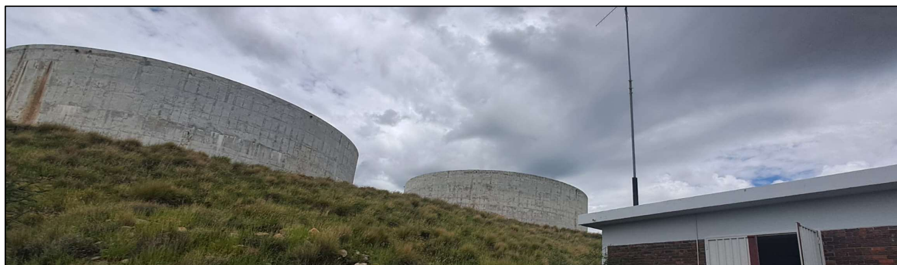
Figure 12: Otjihase 4 000 m 3 reinforced concrete reservoirs.
