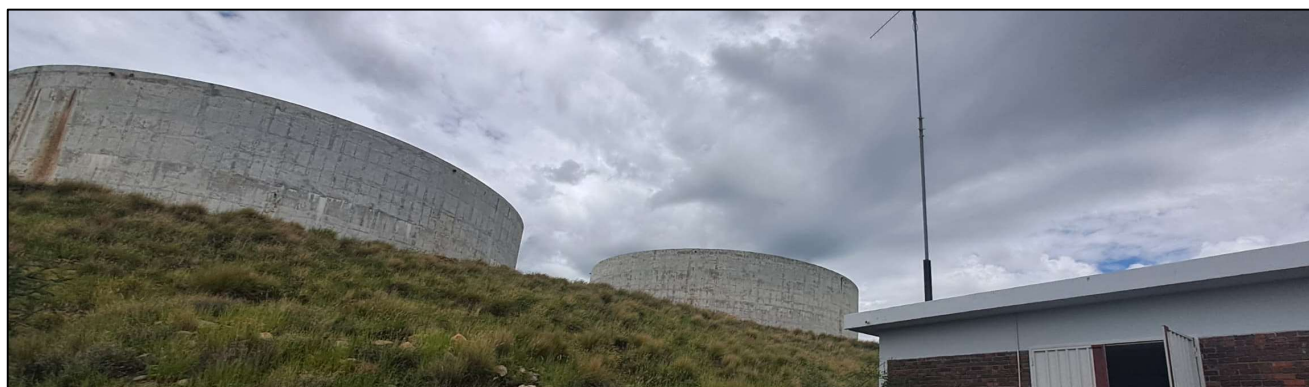
Figure 12: Otjihase 4 000 m 3 reinforced concrete reservoirs.
