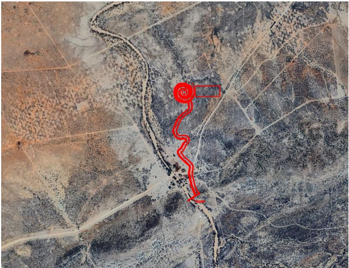
Figure 9. Okawayo River diversion and embankment dam site.
