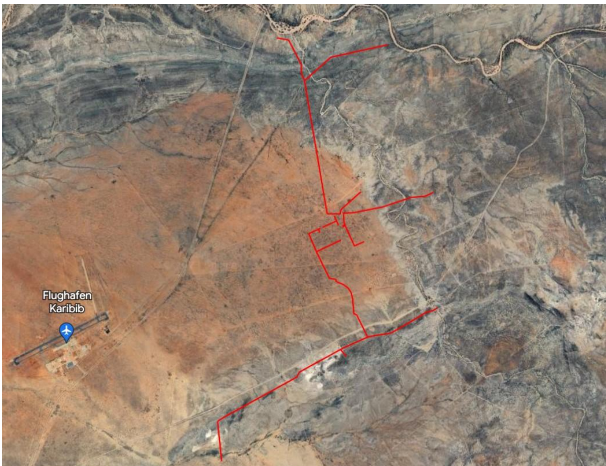
Figure 5. Various 11 kV overhead transmission lines.
