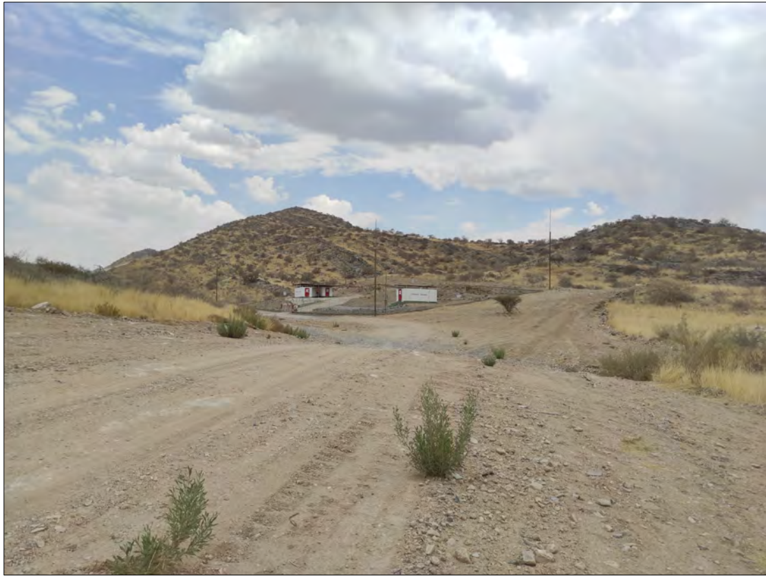
Figure 38 - Second water channel flowing across the road
