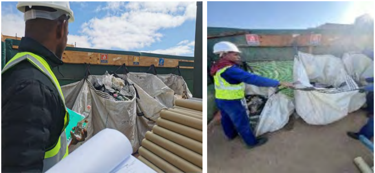
Figure 3 - Solid waste segregation bags used on site during construction
