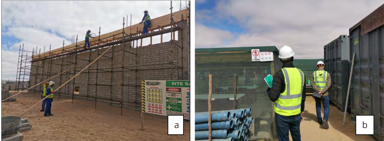
Figure 2 - Construction of Project building (a) and site temporary support structures during construction (b)
