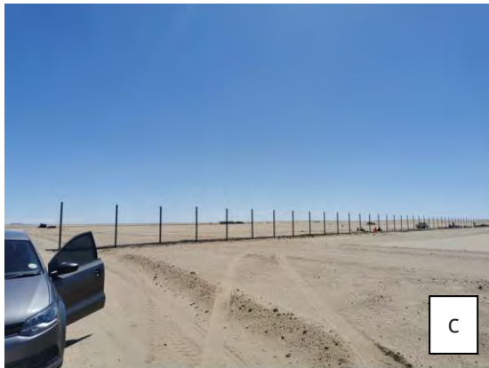
Figure 9 - Serviced fire extinguisher (a), employee wearing the required PPE (b) and meshed fence surrounding the Project footprint (c)
