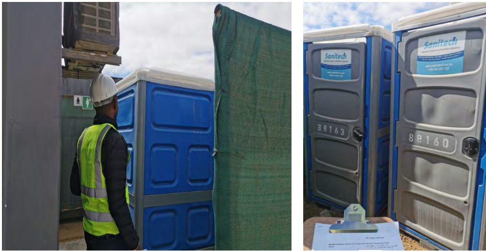
Figure 4 - Portable toilets kept on site for employees and visitors during construction
