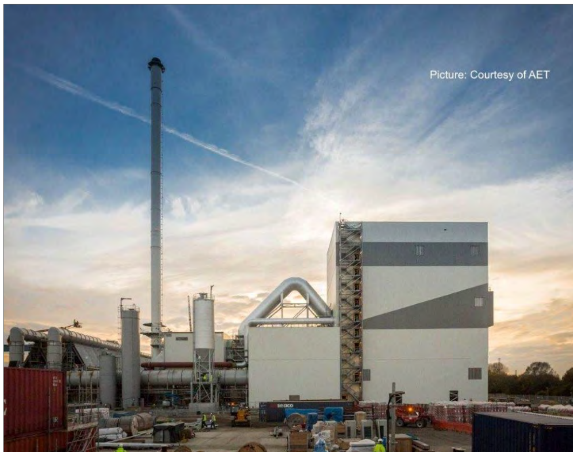
FIGURE 4-13: SIMILAR BIOMASS POWER STATION (TILBURY GREEN 40 MW BIOMASS PLANT IN LONDON)
