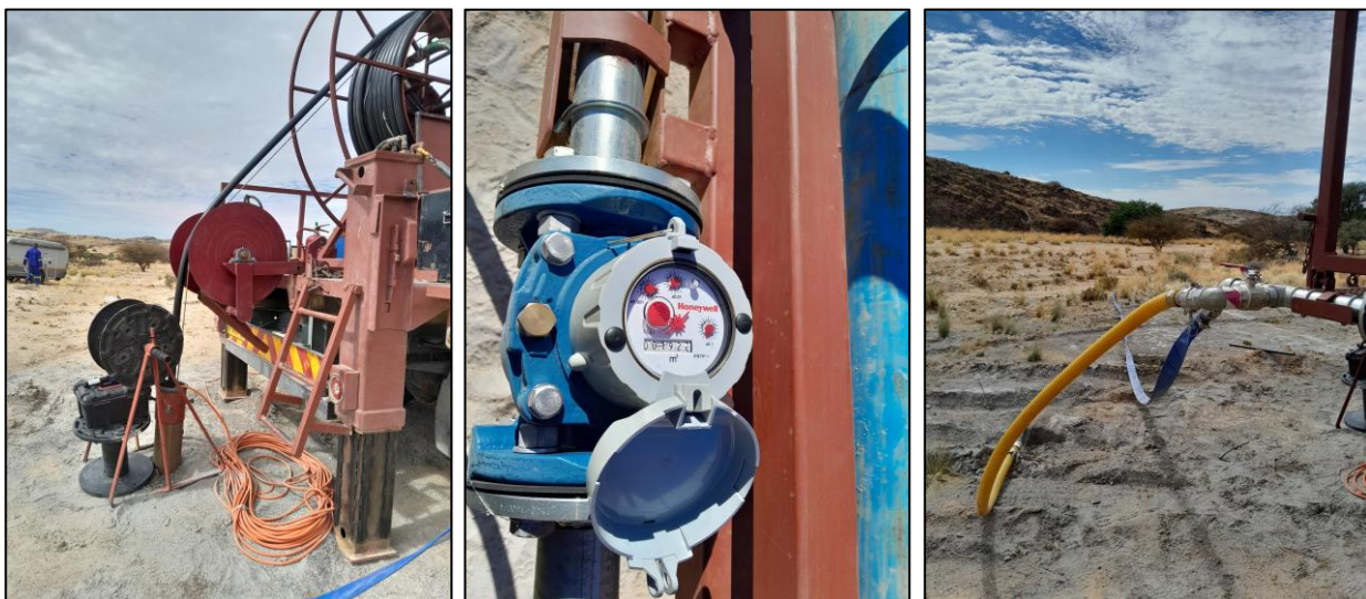
Figure 2 – Test pumping setup at PNNBH_02 and PNNBH_04
